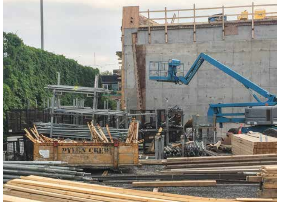
A rear view of one of the two Preston Street rigid bridges waiting to be moved. ALAYNE MCGREGOR/THE BUZZ
