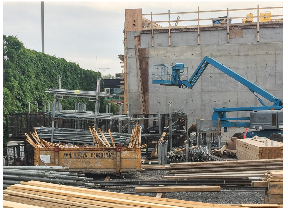
A rear view of one of the two Preston Street rigid bridges waiting to be moved. ALAYNE MCGREGOR/THE BUZZ
