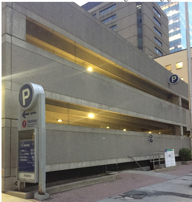
The current grim precast parking garage. ALAYNE MCGREGOR/THE BUZZ
