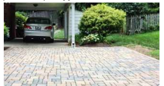
A permeable pavement driveway. RAIN READY OTTAWA
