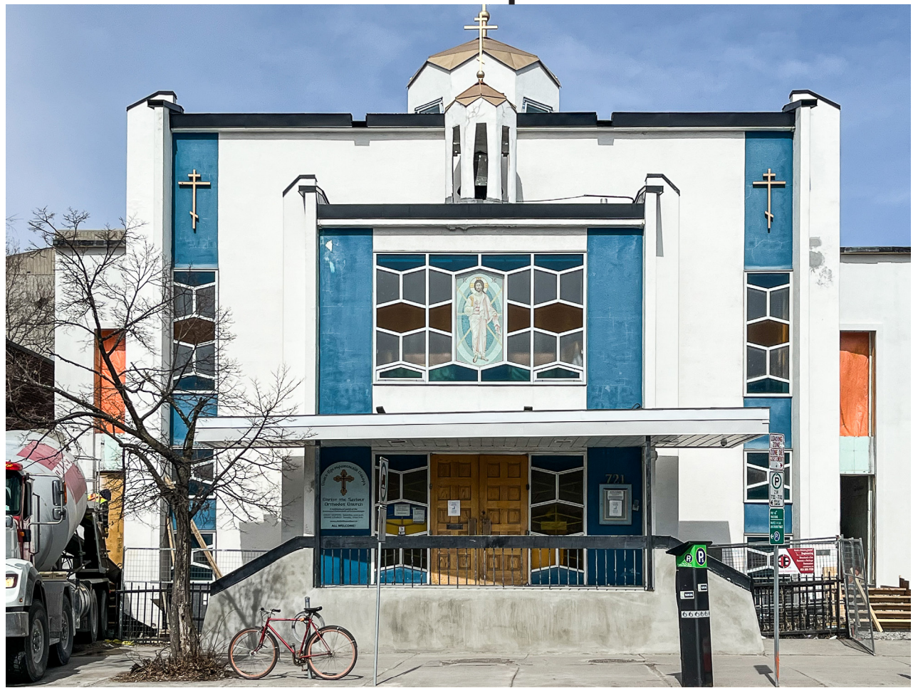
The congregation of Christ the Saviour Orthodox Church chose to stay in Centretown and renovate their building.
