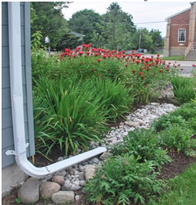
This downspout drains into a rock bed and waters nearby plants, rather than going into the city’s stormwater system. This reduces the need for expensive city water and decreases the risk of flooding. RAIN READY OTTAWA
