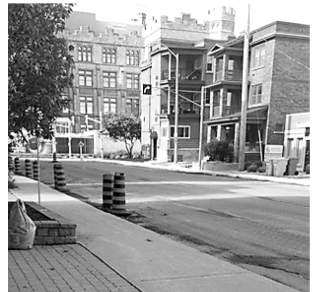
A dangerous section of Metcalfe Street where the curb and the street no longer matched. RYAN LYTHALL/THE BUZZ
