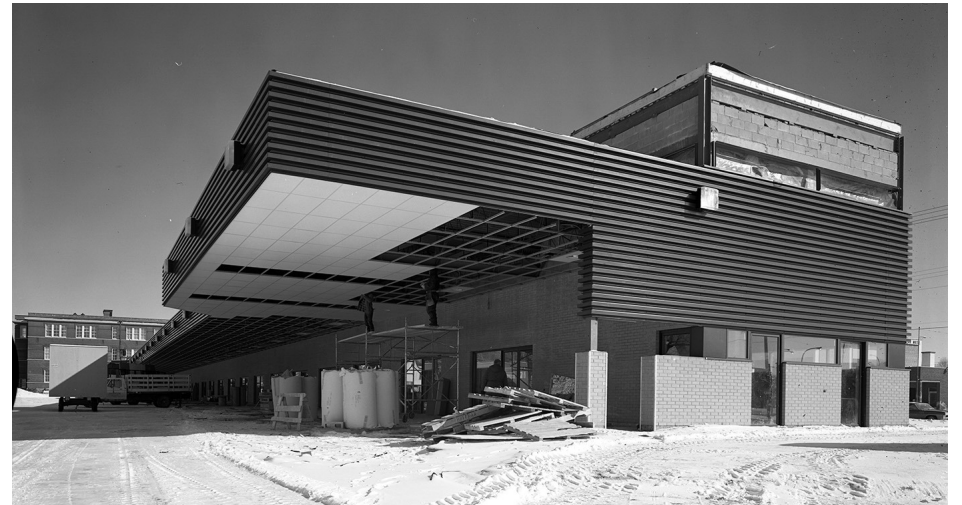
The Voyageur Colonial bus terminal under construction. It opened in 1972. (CMHC)
