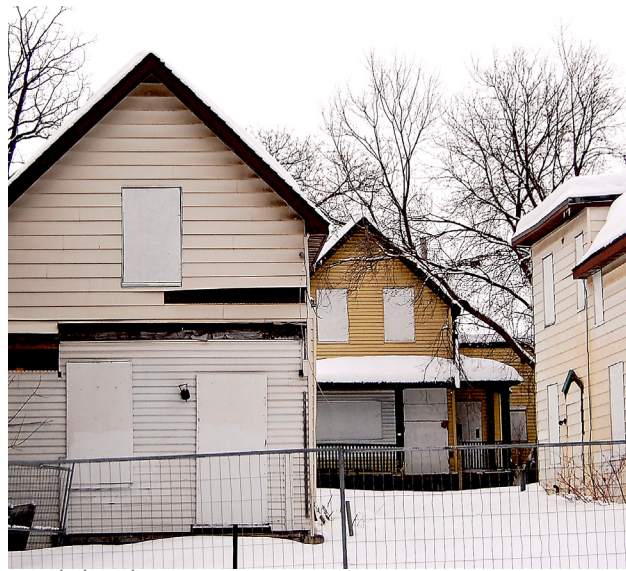
Boarded-up houses in Centretown.
