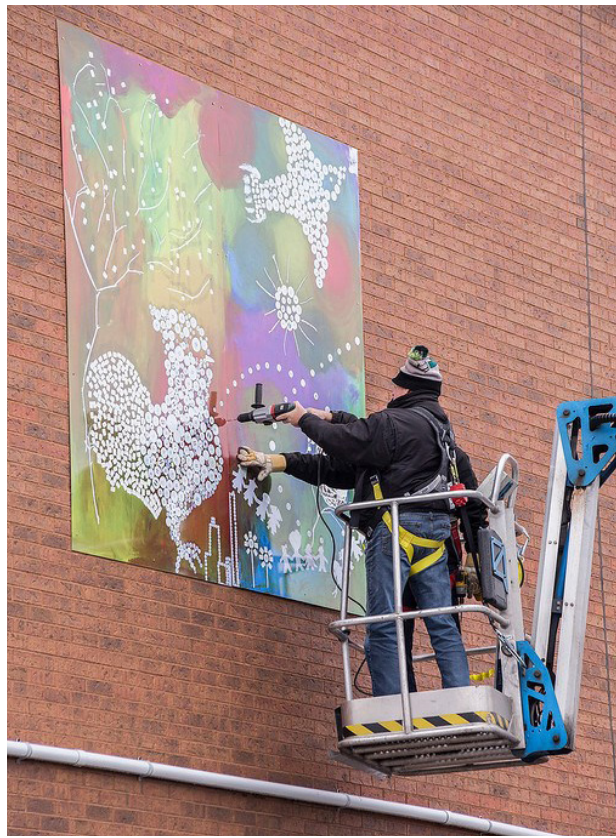
Installing a mural on the school wall. GLASHAN PARENTS COUNCIL
