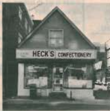
168 O'Connor St/Heck's Variety Store Date of Construction: 1878
